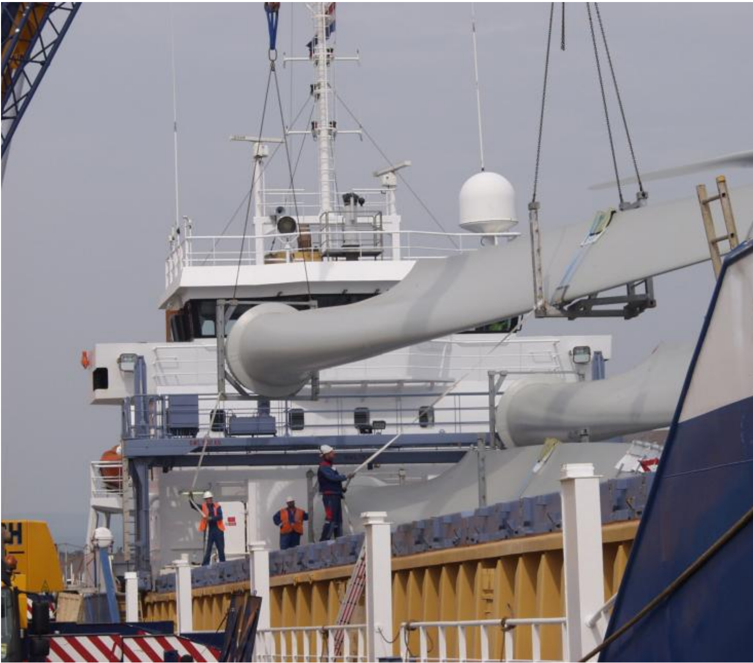
Wind turbine blades being discharged at Avonmouth Dock
